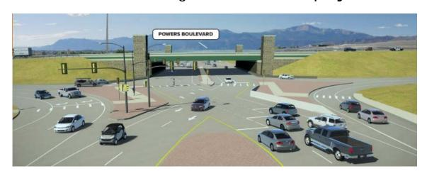
The SH 21 and Research Parkway Interchange project constructs a grade-separated interchange to improve safety and mobility on SH 21 (Powers Blvd) including 3 miles of paving. Adds sidewalks and bike lanes to improve access from an elementary school on the east and middle and high schools on the west.
